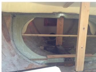
One of the identifying features of an early R19 is a solid bulkhead under the foredeck. The forepeak space was filled with Styrofoam blown in through two holes drilled in the foredeck. Needless to say, the foam soaked up water, so I cut a hole for a 10" port low in the bilge, and a large hole for a watertight, locking hatch higher up. Now I can put some G10 under the forestay fitting, and install new mooring cleats in the waterways, in the area where the chocks used to be.
